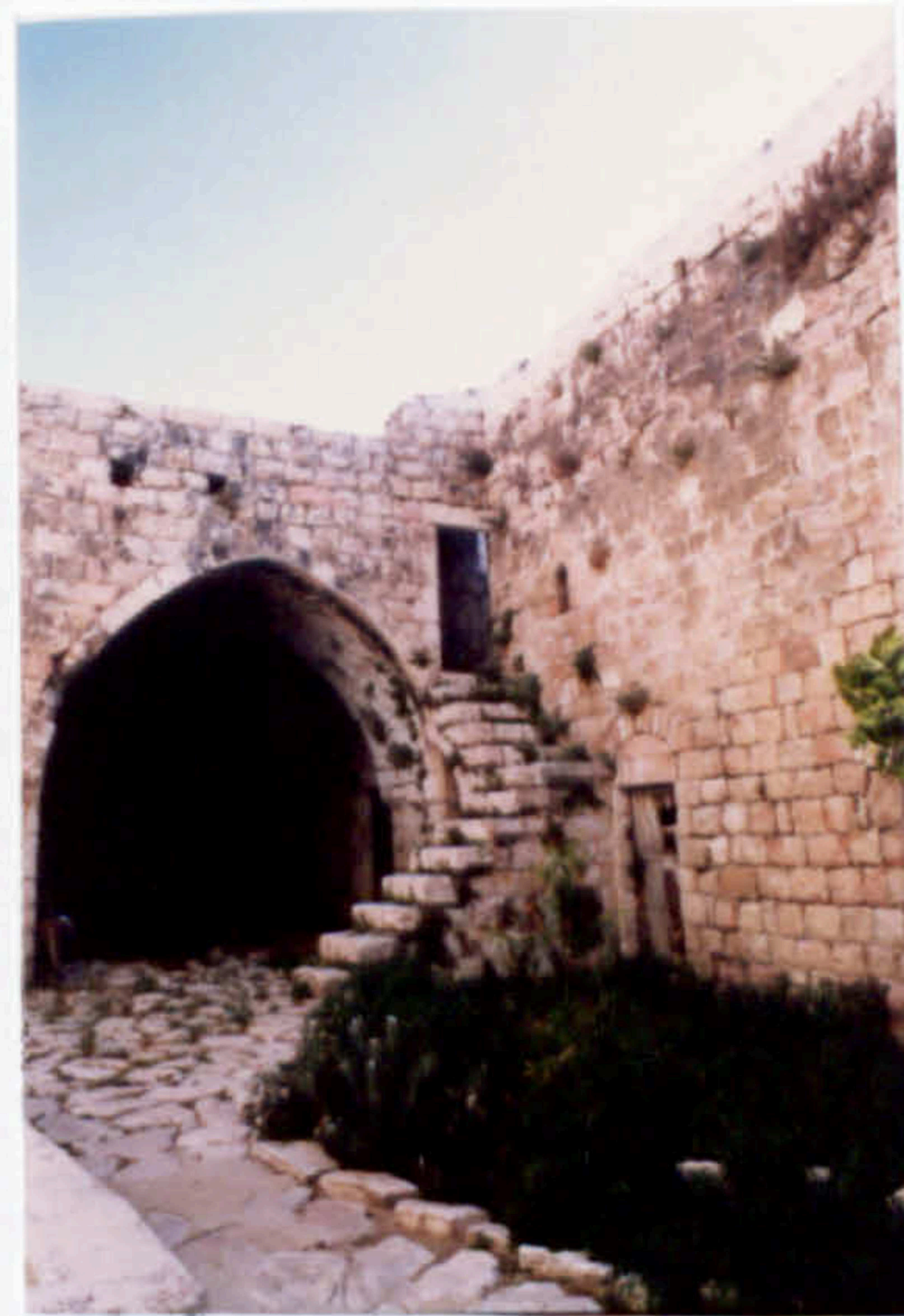
Stairs to elevated rooms
