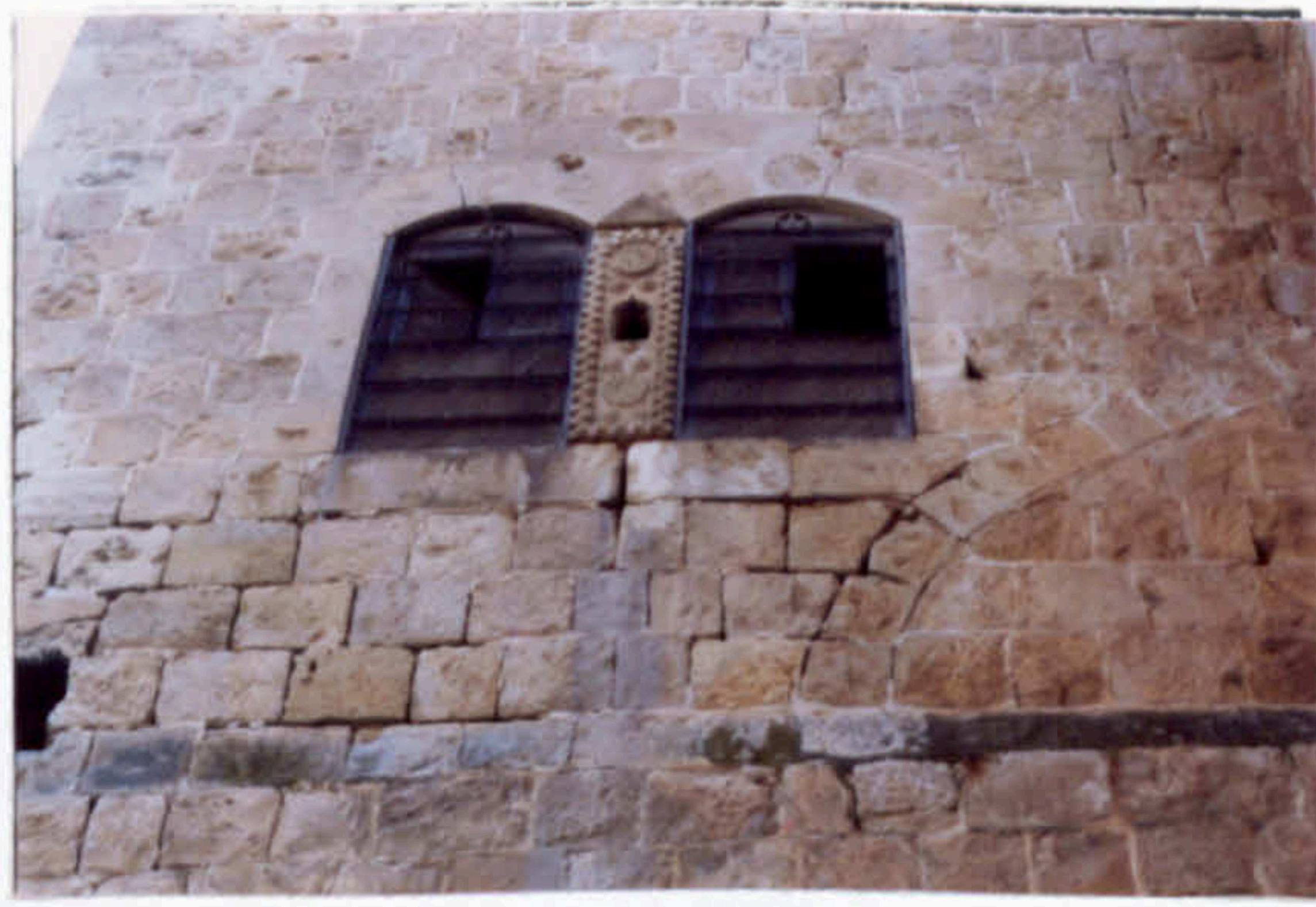
Lattice wood windows
