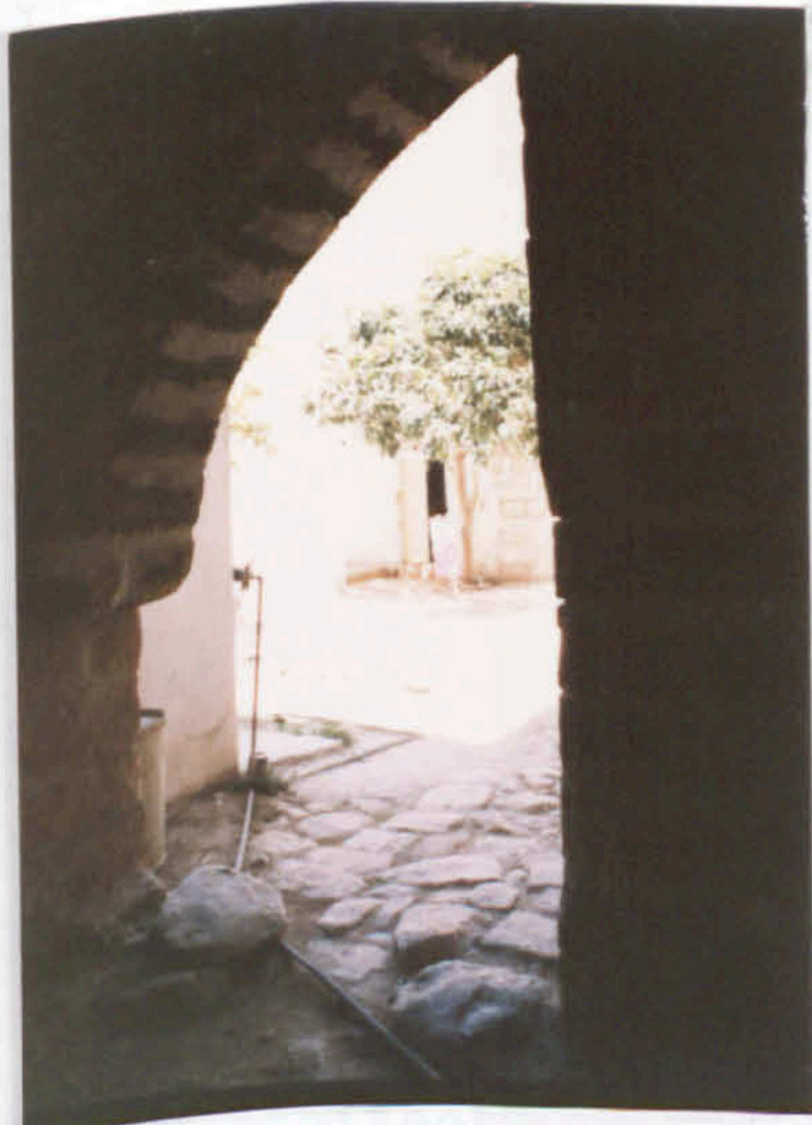
court from entry vestibule
