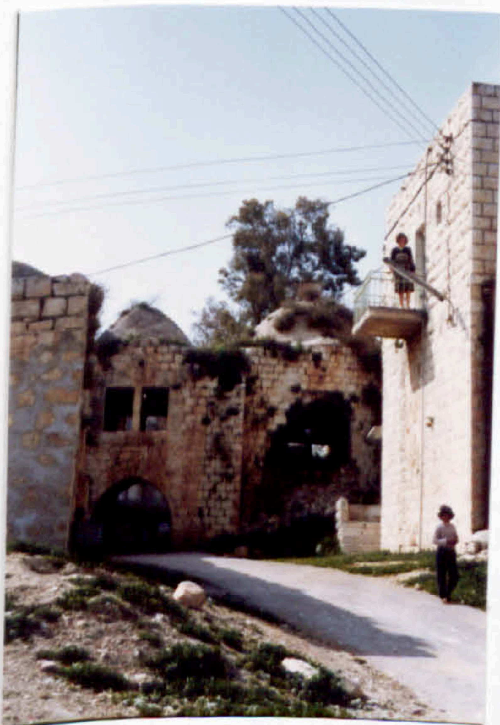
The guest-house in deterioration
