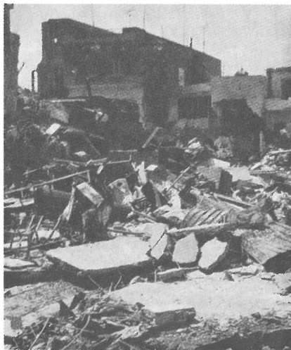
Destruction in Sabra
